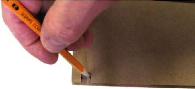
Marking for a new hole the same distance from the edge, but centered between the marks
